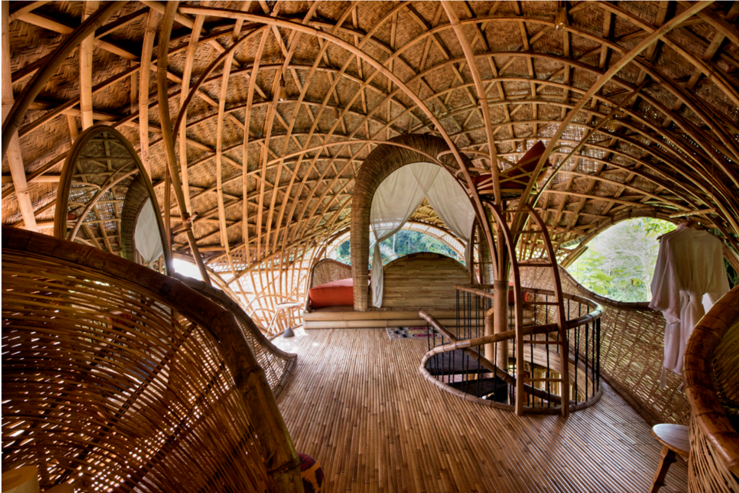
Riverbend House by IBUKU at Bambu Indah, using splits bundles
