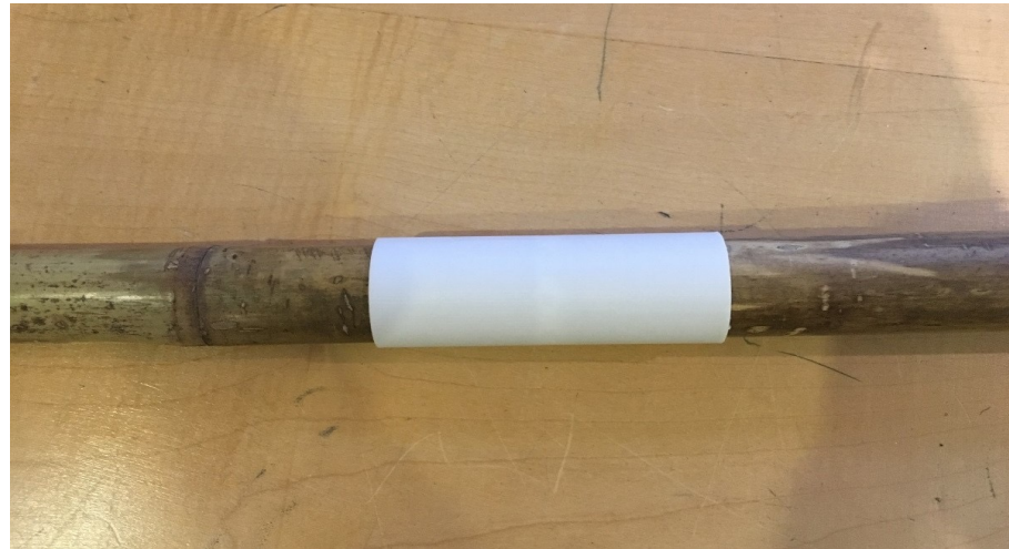
Typical detail to create continuity between the poles in the gridshell.
